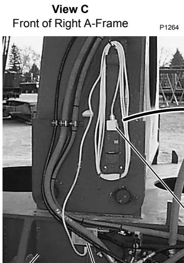
View C Front of Right A-Frame Counterweight Tray Junction Box
